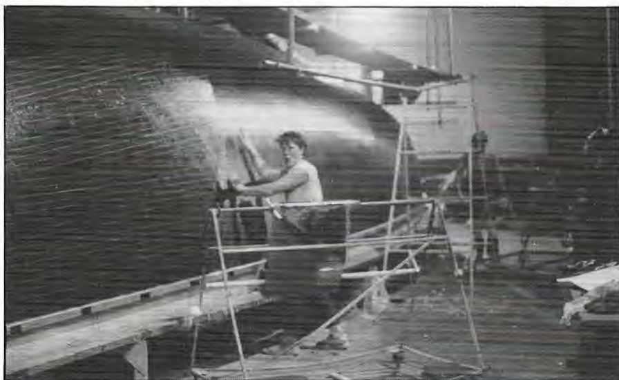
LAYING the inner core of the hull of WINDWARD PASSAGE II — "the most advanced boat ever built".
