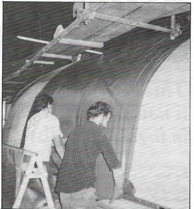
BUILDING shots of WINDWARD PASSAGE II at John McConaghy Boatbuilders in Sydney. ABOVE: The plugs for the hull and deck. RIGHT: Laying up the first layer of carbon fibre and kevlar. BELOW: Extra reinforcing in high load and slam areas of the 80-foot hull.
