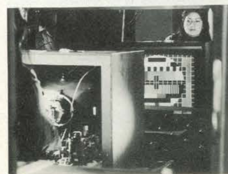
Adjustment of a television receiver during manufacture by AWA.
