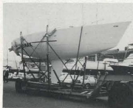
MAD MAX — KZ 296 LOA 40' 2" / 12.9 m IOR 30.5 Construction: Kevlar/Divinycell Date: 1985 Owner/Skipper: Chris Beckett Designer: Davidson NEW ZEALAND 'B'
